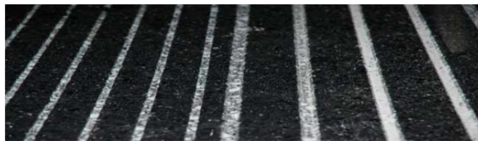
Figure 3. Standard (Left) and Trapezoidal (Right) Grooves Side by Side
