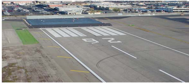
Figure 4. Aerial photo showing the original, materially-designed arrestor bed system installed off Runway 26 at Burbank Airport, Burbank, California
