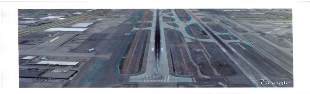
Figure 1. Excessive rubber build-up on the runway
