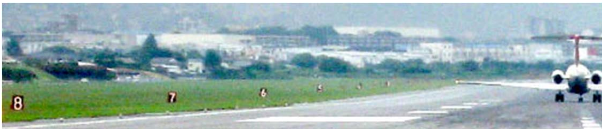
Figure 2. Distance remaining signs along a runway; close-up view of an individual installation
